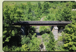
Railroad Trestle This historic 160' long, 60' high trestle, with its monumental limestone piers, was built in 1880s to span McCarn Creek.
